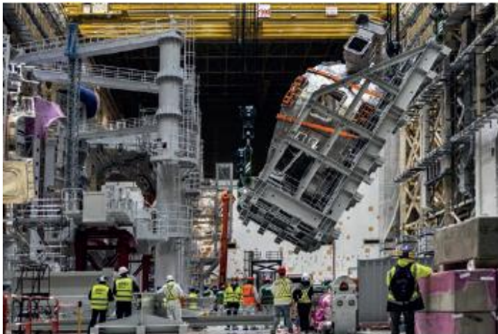
Moving upright a 440 t sector of the vacuum vessel, to bring it to the assembling tool on the left of the image (Korean sector, 11.12.2021). © ITER.
